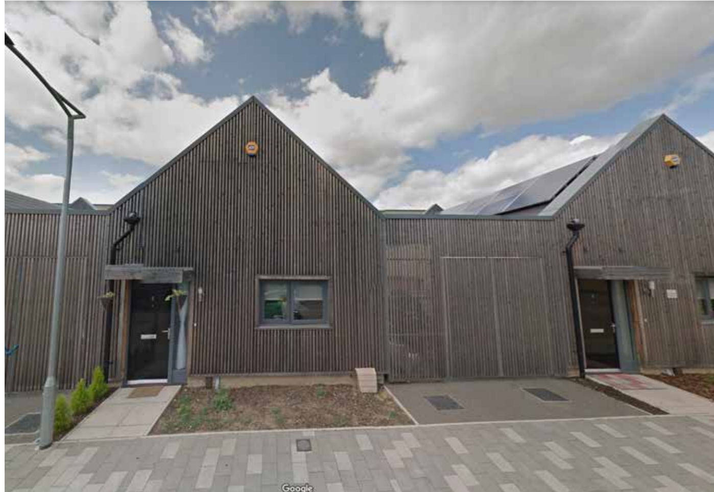
TYPICAL AS-BUILT TIMBER ELEVATION TYPE CF
